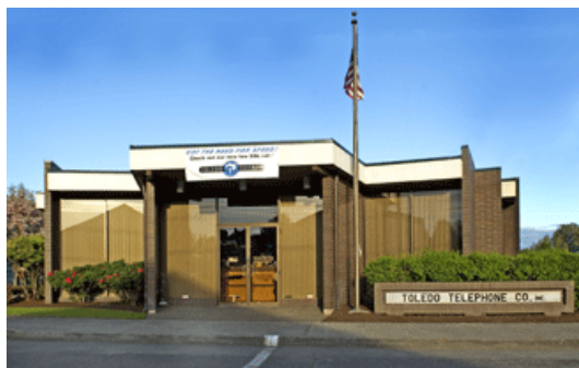
Toledo Telephone Central Office
